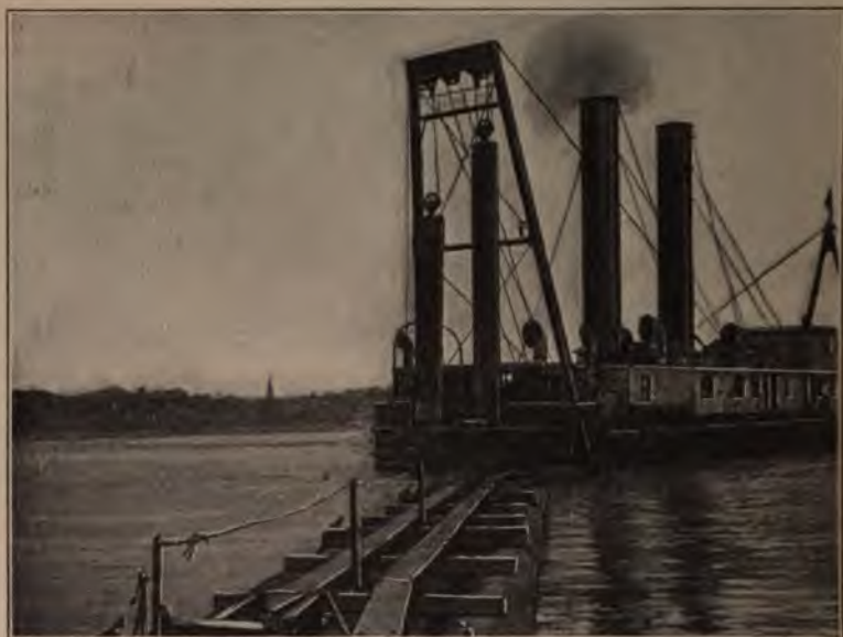
Rear View of Hydraulic Dredge Operating in Lincoln Park, Chicago. Figure 113.
